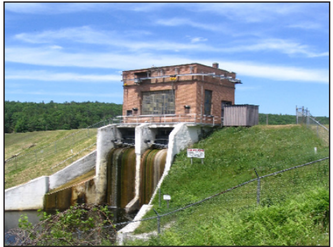
Boardman River Dam
